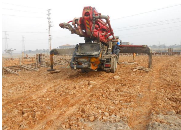
Factory construction site
