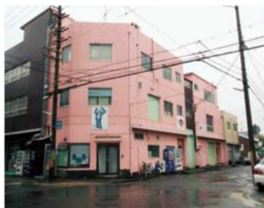
Headquarters front view
