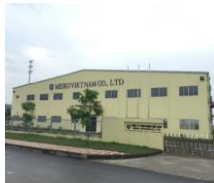
Full view of the Vietnam plant
