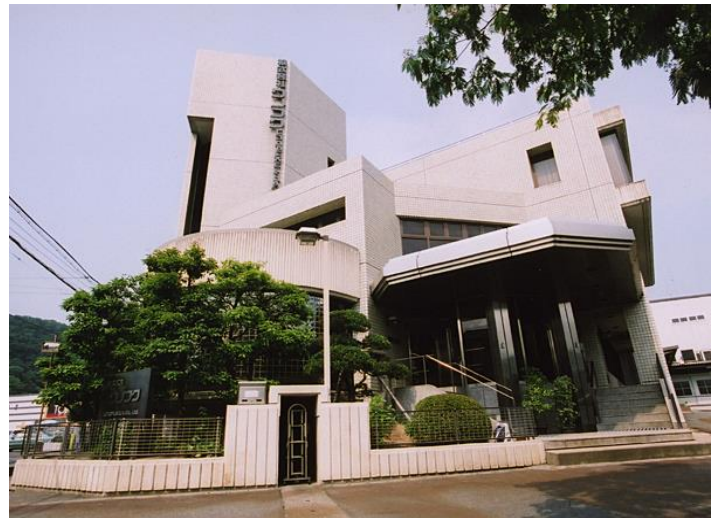
Headquarters front view
